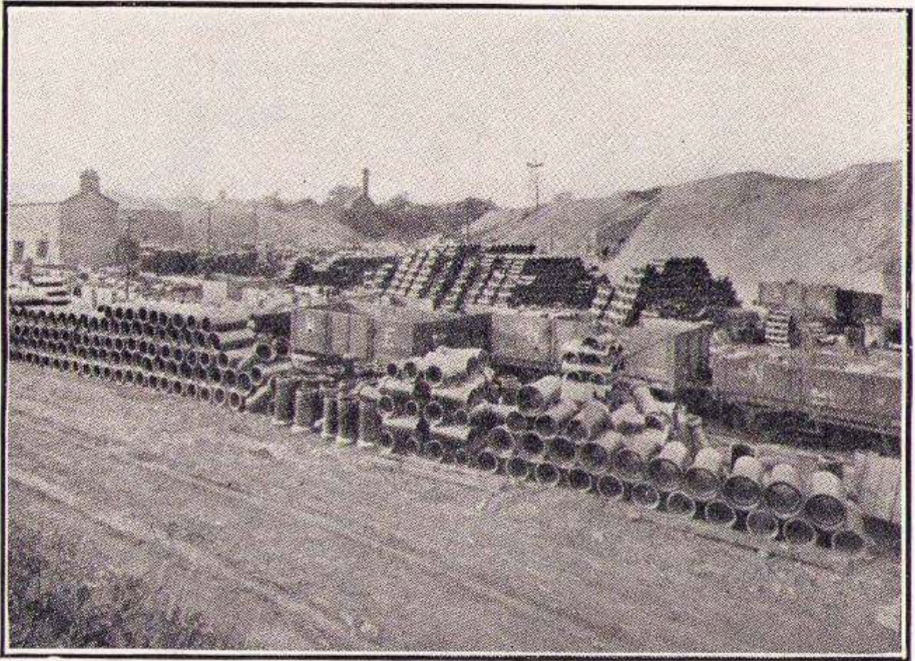
One of the Loading Decks for Transport
